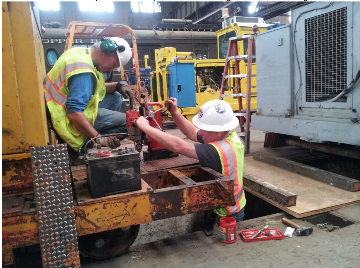
Ed and Steve having too much fun using the mag-drill to fasten the deck plates to the Kalamazoo
