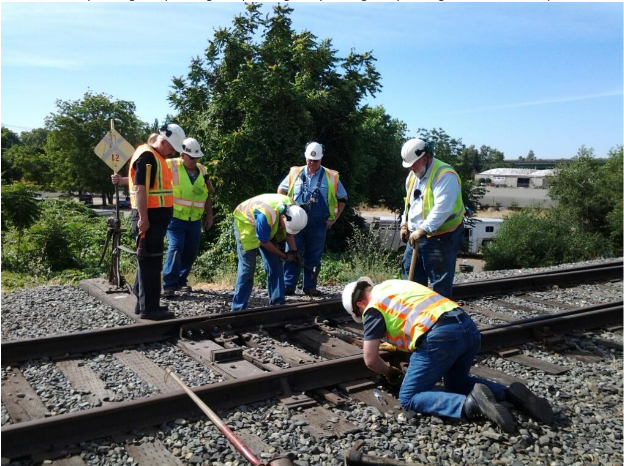
Fred, Harry, Steve, Chris, Frank, and Ed mitigating the defect at Switch 12
